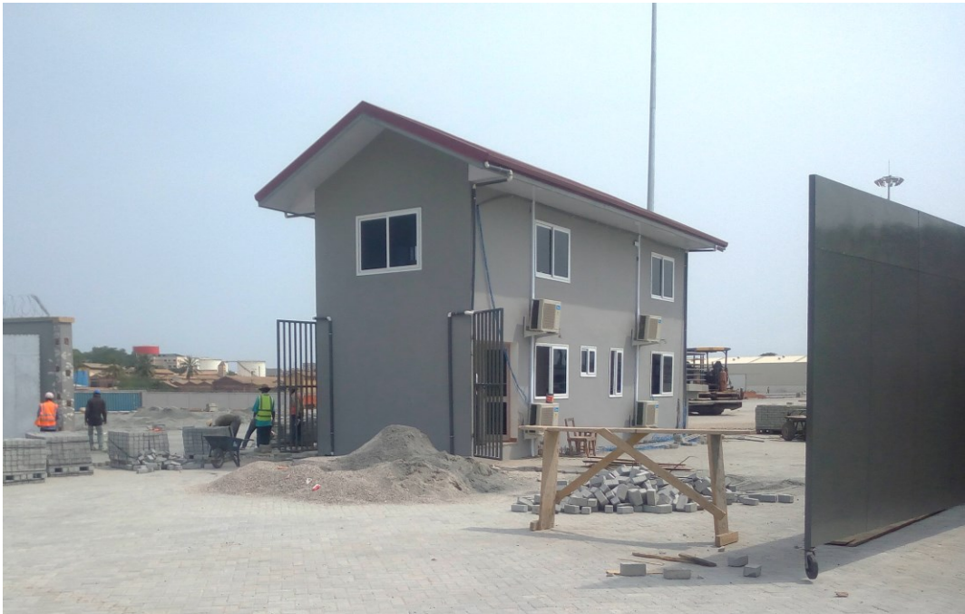
Figure 2-10: Reception facility under construction at entrance of container handling area
