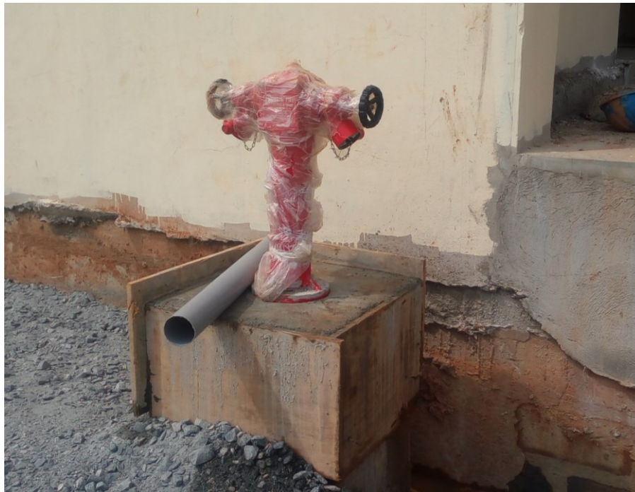
Figure 2-3: Fire hydrants been installed at TACOTEL
