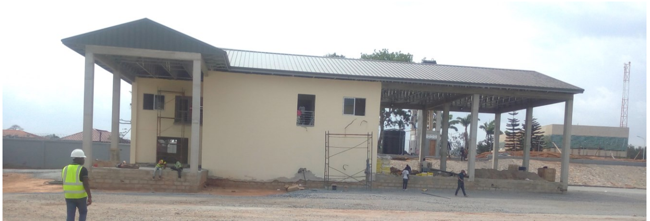
Figure 2-9: Mechanical shop (equipment repair area) under construction
